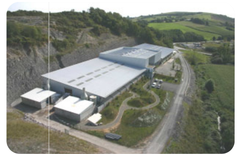
Covered composting facility
